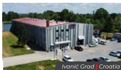
Roto Group Headquarters
